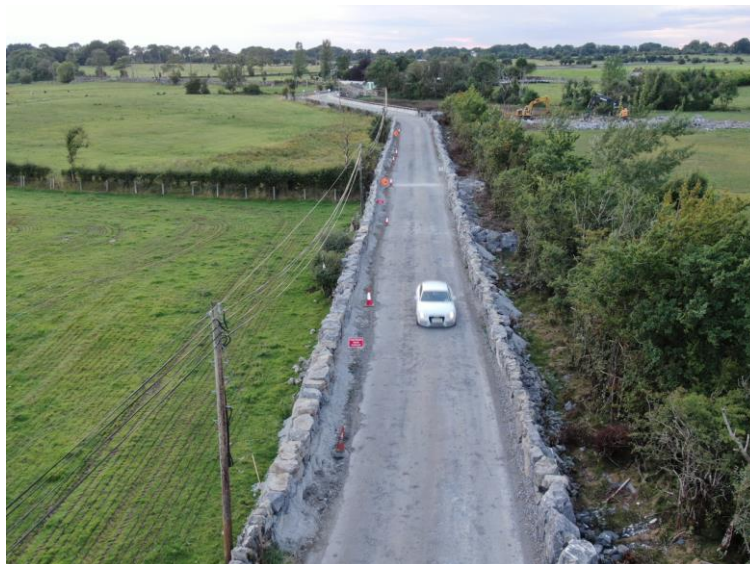
September 2022 – Rock armour works completed. Road raising works pending.
