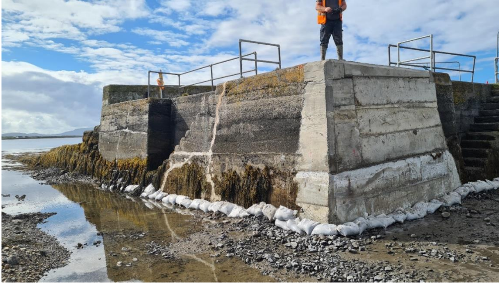
Pictures above show Blackweir Pier before and after works undertaken
