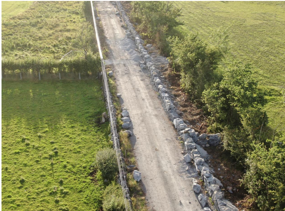
Rock armour walls under construction – August 2022
