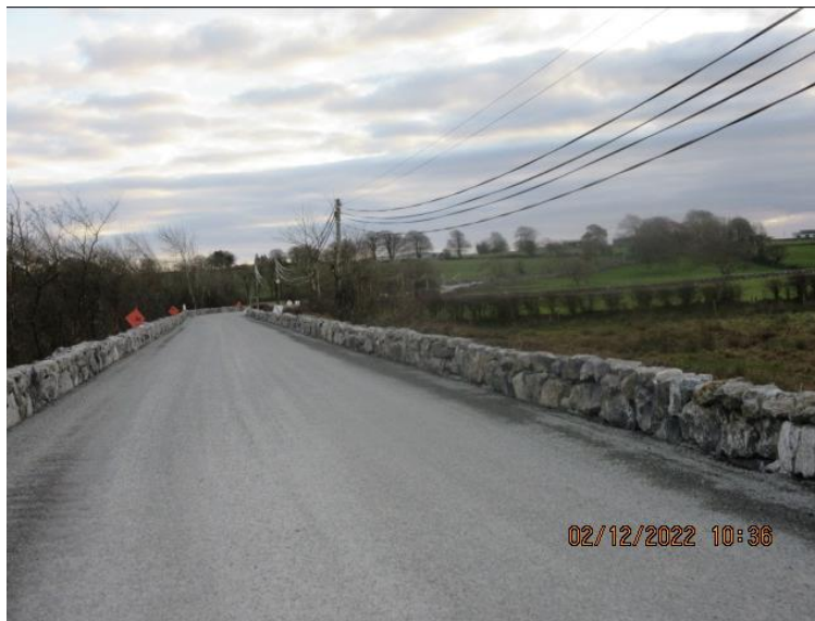
December 2022 – Road raising and surface dressing works completed
