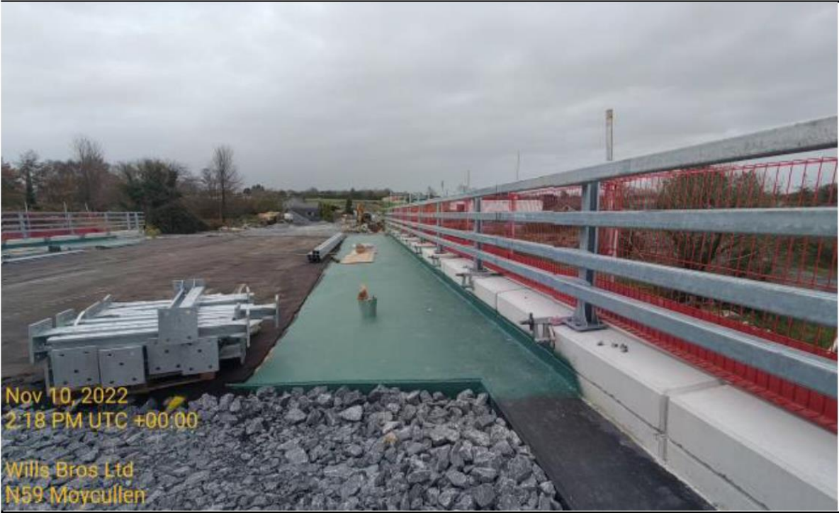
Parapet Railing Installation to ST04 Ballyquirke Canal Overbridge
