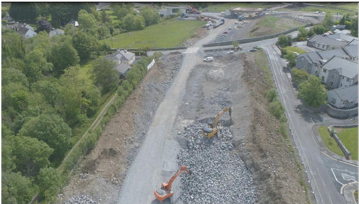
Rock Breaking at Cut 02 Adjacent Knockferry Road
