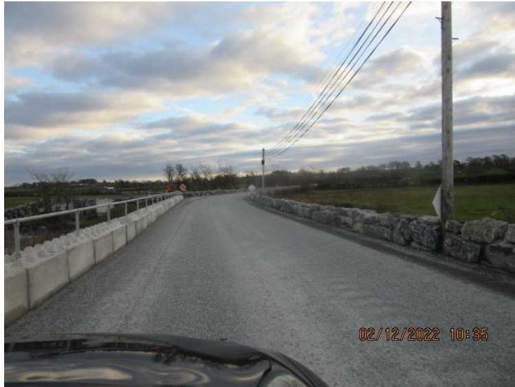
December 2022 – Road raising, and surface dressing works completed
